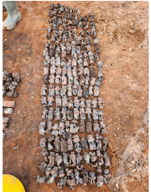
Image showing detonated 2-inch Mortars found during excavation works in Nottinghamshire.
